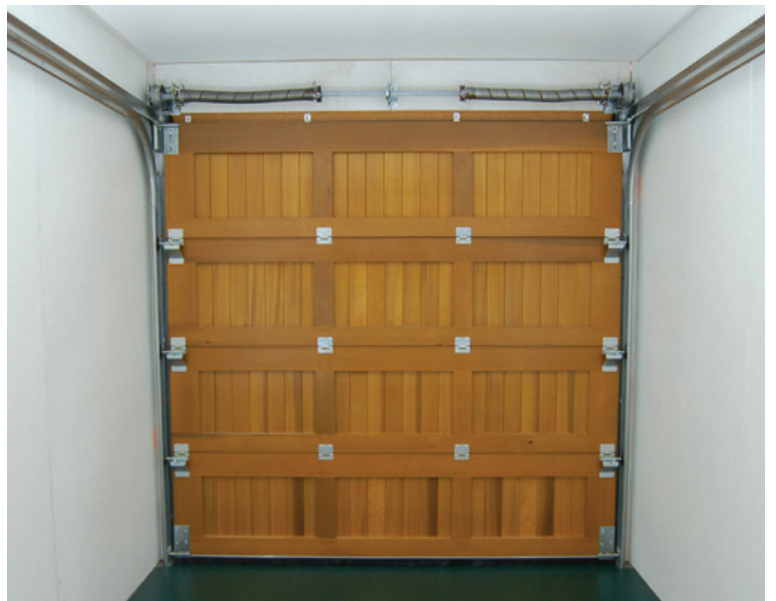
Inside view of sectional door with front mounted spring
