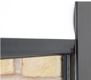
Brush strips reduce draughts and the bottom seal keeps out wind blown debris.
